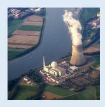
The 1200 MWe Leibstadt Nuclear Power Plant in Switzerland. The boiling water reactor (BWR), located inside the dome capped cylindrical structure, is dwarfed in size by its cooling tower. The station produces a yearly average of 25 million kilowatt-hours per day, sufficient to power a city the size of Boston. By Hansueli Krapf - Own work: Hansueli Krapf (User Simisa (talk · contribs)), CC BY-SA 3.0, https://commons.wikimedia.org/w/index.php?curid=110649554
